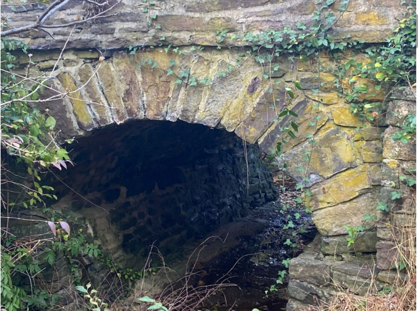
Photo 5: Federal Twist Road stone-arch bridge, west (upstream) side, view facing east showing the keystone and inset panel.
