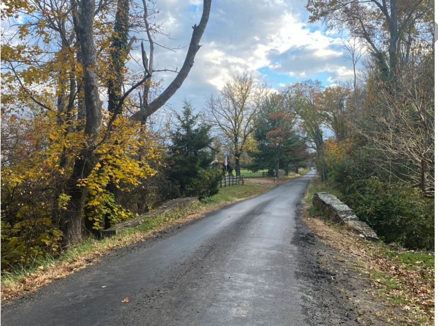
Photo 3: Federal Twist Road at the bridge. View facing south showing the roadway.
